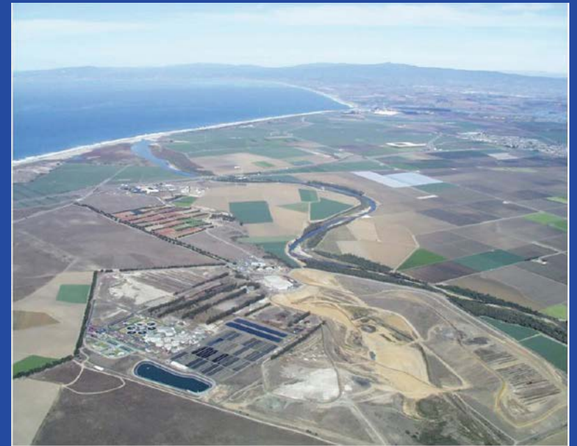
Salinas Valley Reclamation Project
